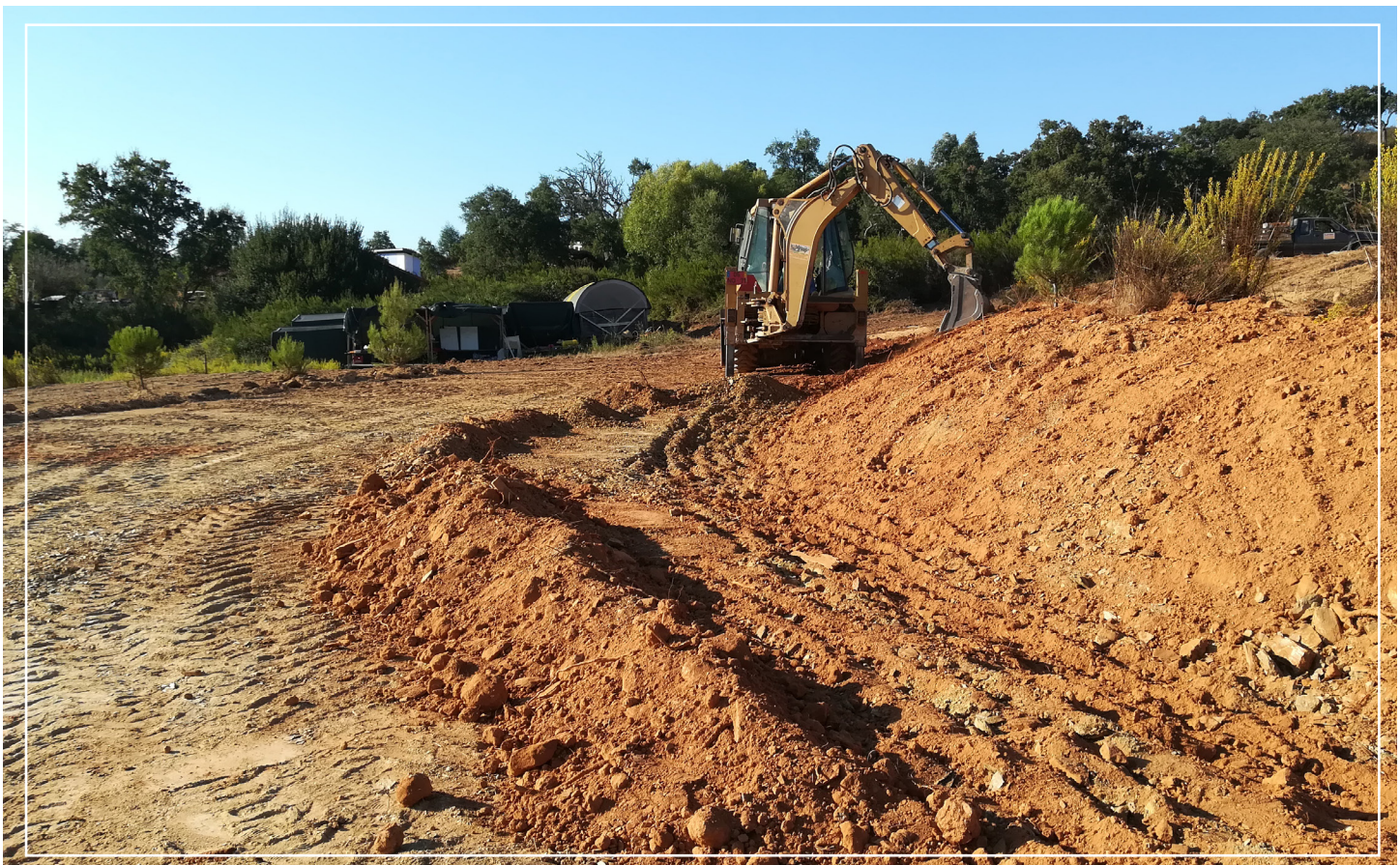
Photo 6. drainage ditch on T1
