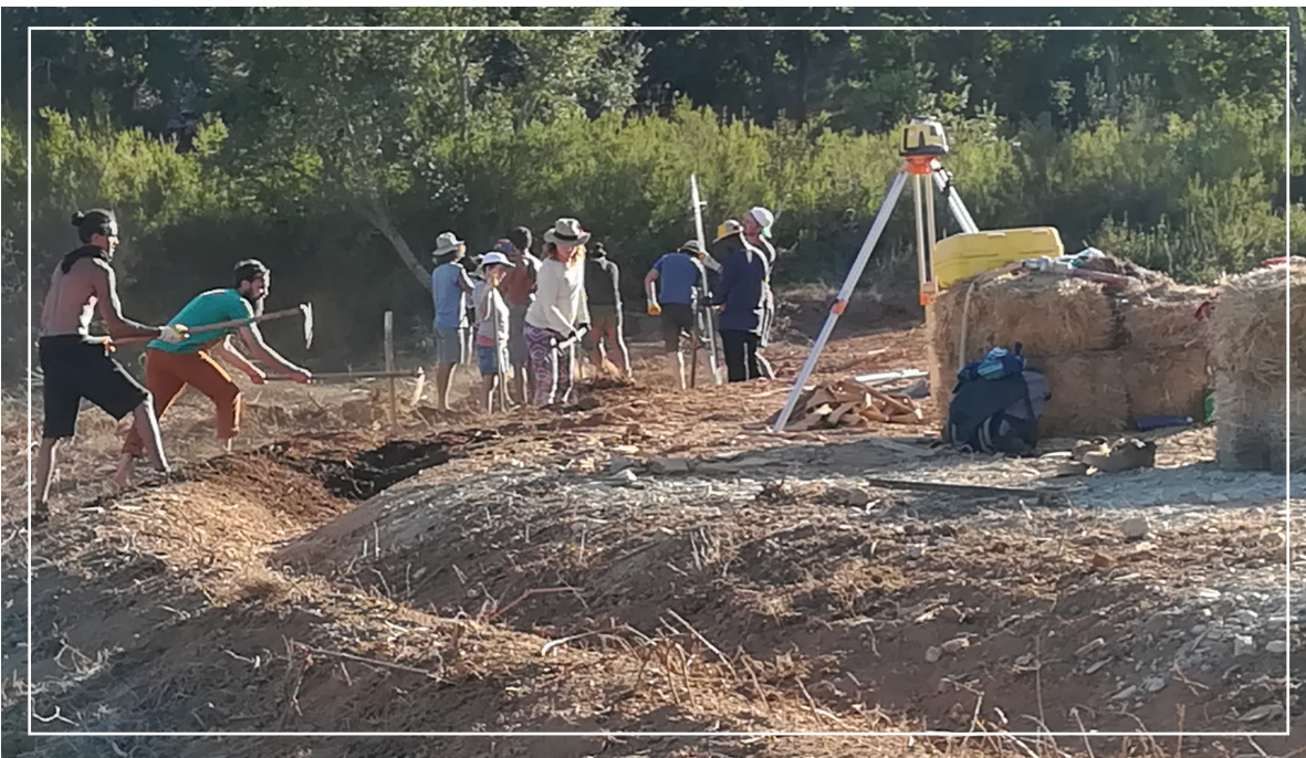
Photo 2. swale along T3
