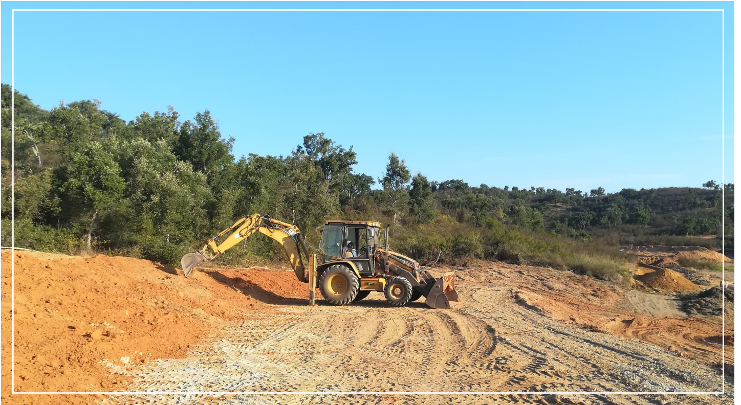
Photo 12. construction of T2
