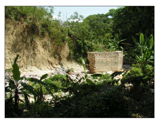
Issue: Destroyed river embankment in same ravine (heavy seasonal flooding) Recommendation: Water retention upstream, infiltration of water also in settlement areas, avoid total sealing of soils
